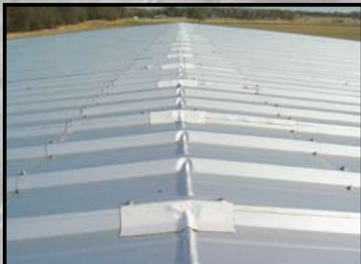
Works on Metal Roofs
